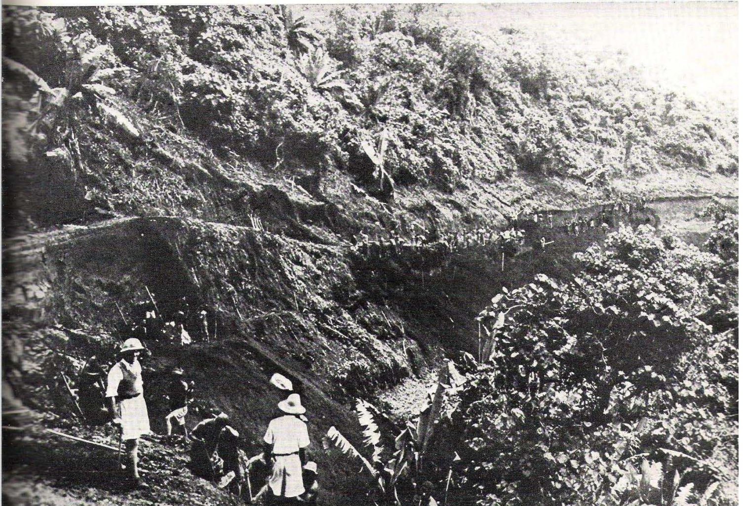
Belgian engineers turned trails into highways.
