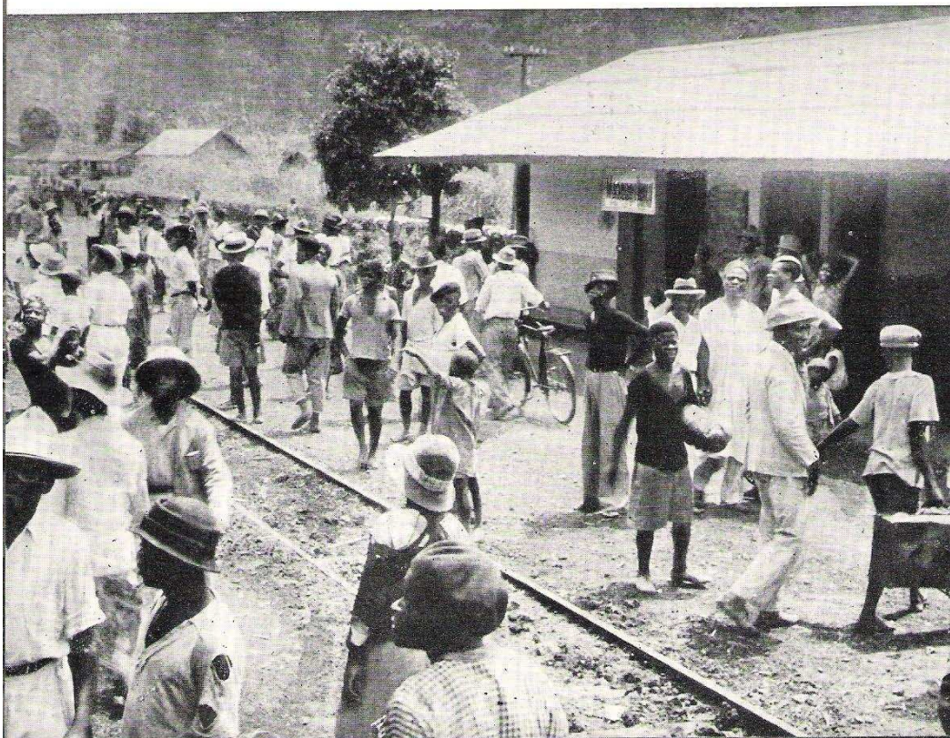
A small railroad station.
